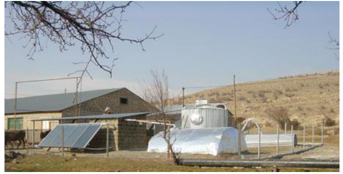
Figure 15. Solar integrated 25m 3 digester based bio-gas pilot project at farms in Arzni village
