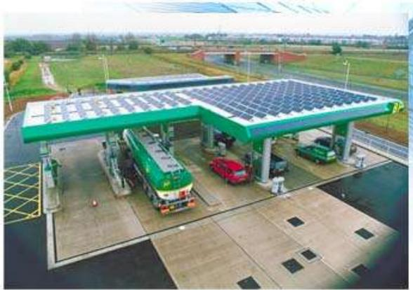
Fig. 5.9. Use of PV system at gas-filling station.
