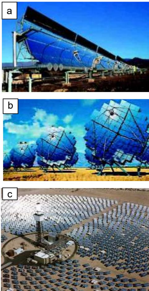
Fig. 4.2. Solar thermal parabolic trough power plant (a), parabolic dish power plant (b) and solar tower power plant (c)
