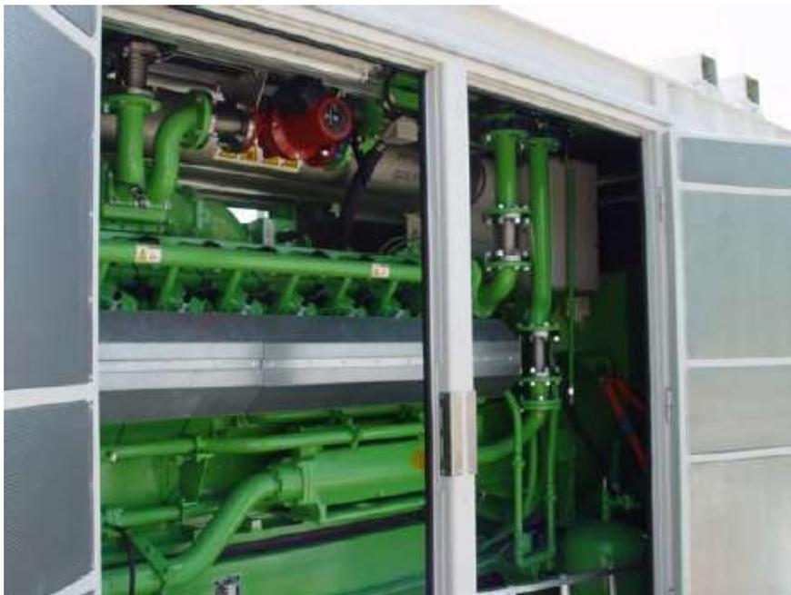
Fig. 7.6. Gas engine installed at Lusakert Biogas Plant
