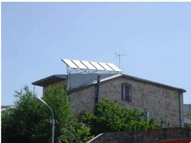
Fig. 6.12. Solar water heating system. Total area of solar collectors is 13m<sup>2</sup> (2006)
