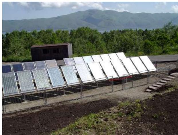
Fig. 6.13. Solar water heating system installed in the yard of Vasgenian theological seminary (Sevan) [18]
