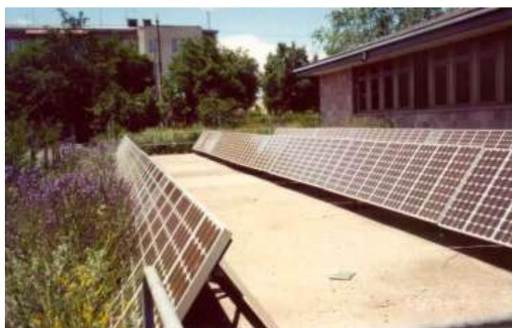
Fig. 6.4. 7.5 kW PV station in t. Gyumri
