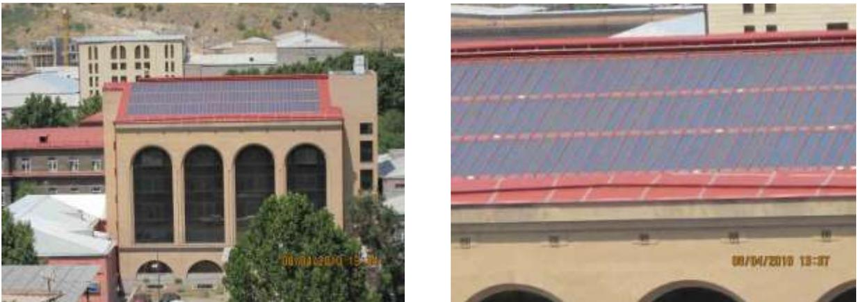
Fig. 6.9. 10 kW solar photovoltaic station installed at Armenian-American Health Center
