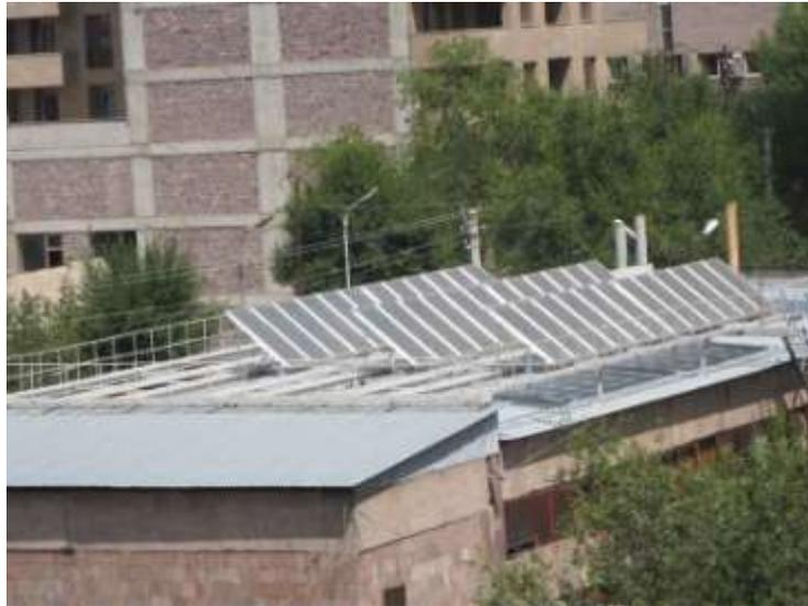
Fig. 6.11. Solar water heating system integrated with boiler house.
